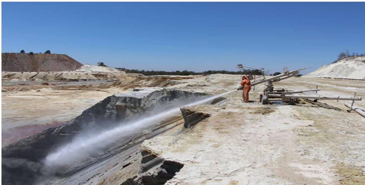
Figure 3: Reclamation of a slimes dam for re-processing
