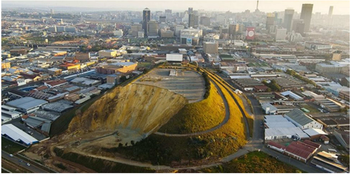
Figure 6: Sand heap gold mine tailings
