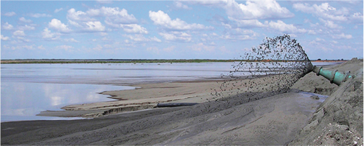
Figure 8: Slimes dam construction using a hydro-cyclone
